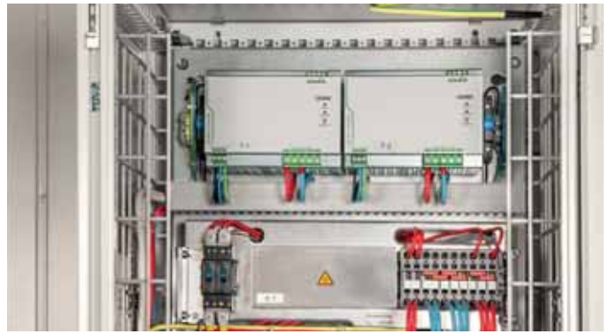
Redundant power supply with diode de-coupling
